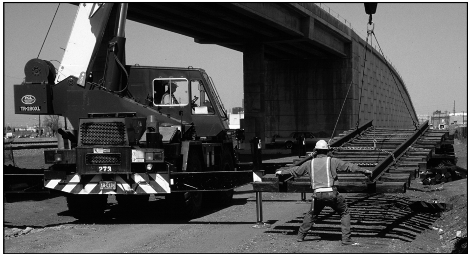
The relocated Joint Line continues to take shape. RTD's Southwest Corridor line climbs the Iowa Flyover allowing the BNSF and Union Pacific to continue serving customers on the Iowa Spur in the vicinity of Evans Ave. That spur's trackage was lifted into place under the flyover March 23, 1999. – Photo © Chip Sherman.
